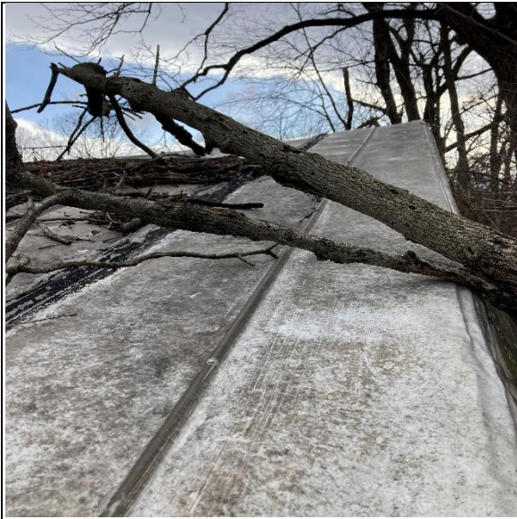
Silver roof coating on shed
