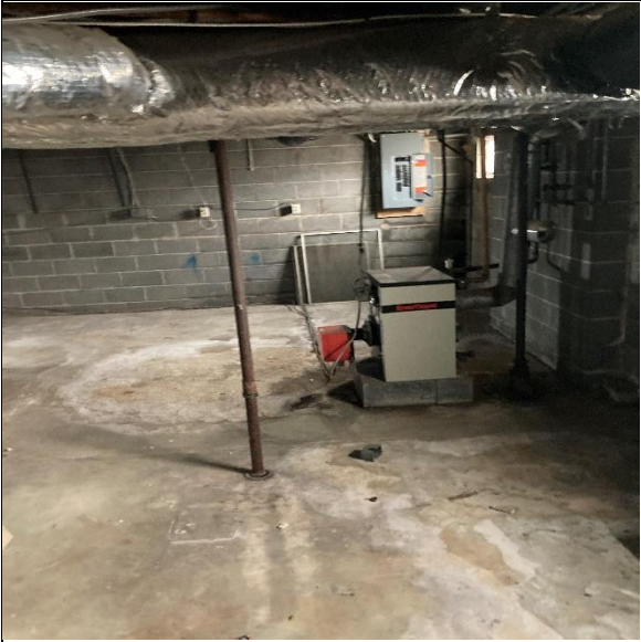
Basement flue mud
