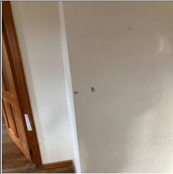
Drywall/joint compound throughout (TRACE)
