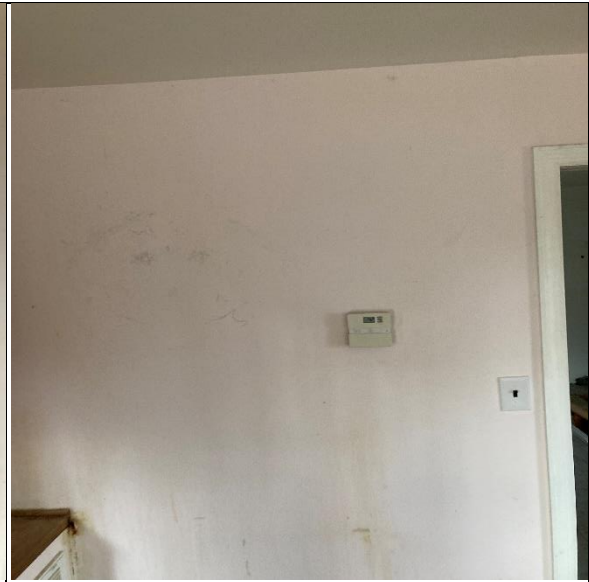
Drywall/joint compound throughout (TRACE)
