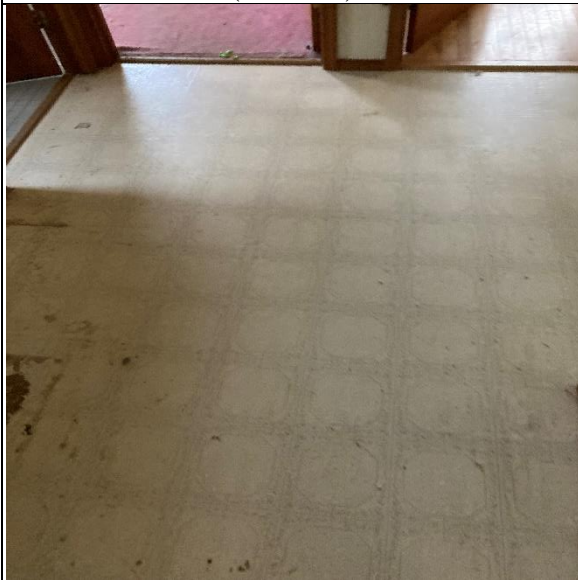
Off white sheet flooring in laundry area
