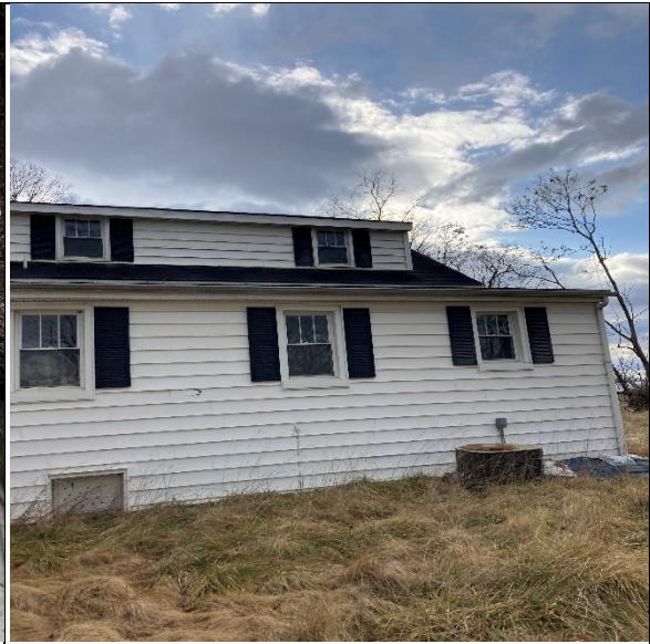
Black asphalt shingles and felt paper
