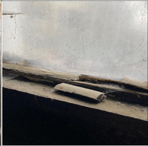
Metal frame window glazing in basement
