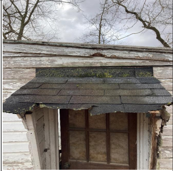
Black asphalt roofing at shed entry
