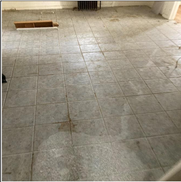
Ceramic tile and grout in kitchen
