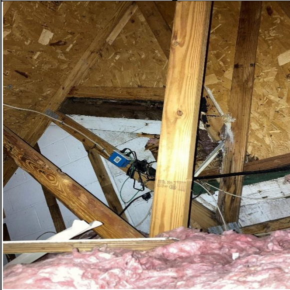
Attic area with fiberglass insulation
