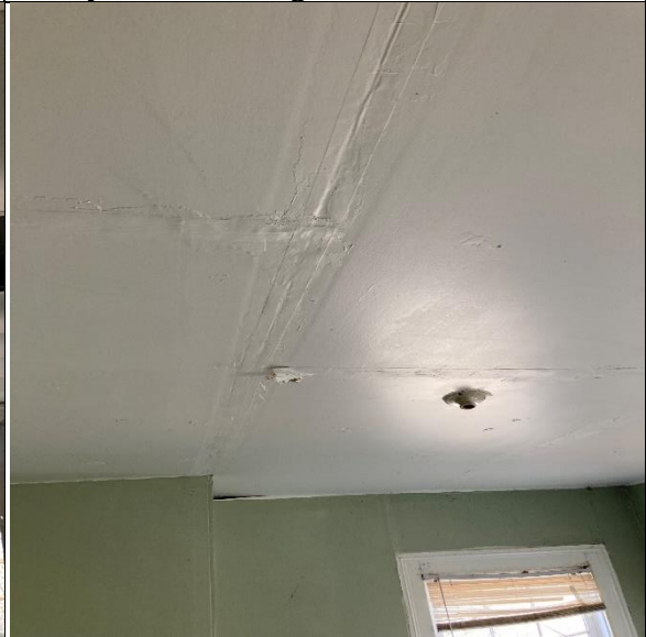
Drywall/joint compound on 2 nd floor
