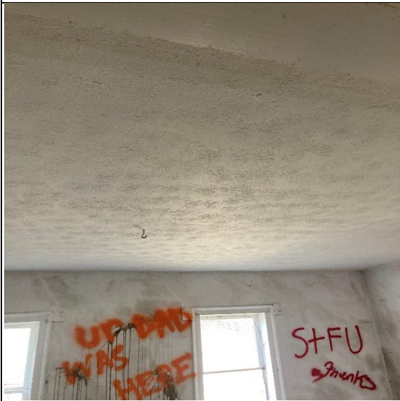
Textured ceiling material in living room area
