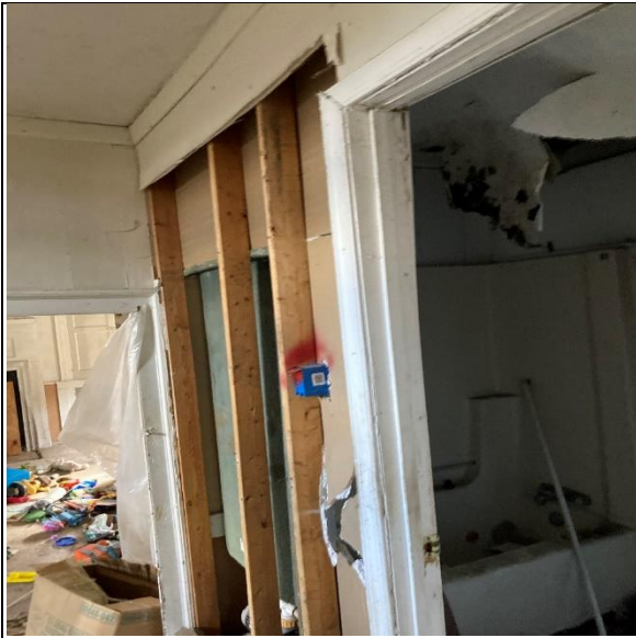
Drywall/joint compound on 1 st floor
