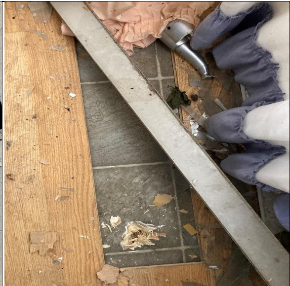
Gray sheet flooring in 2 nd floor bathroom
